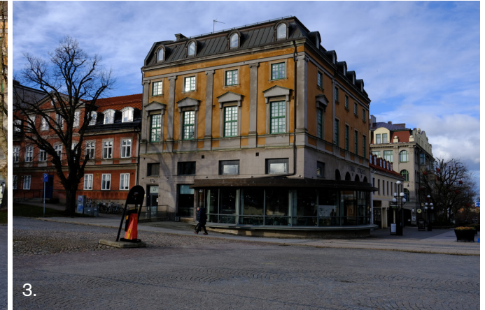
Magistraten 16 Built in 1901 in an Art Nouveau/Neo Rococo style. Rebuilt in the 1920's in a Neo Baroque style. Minor additions towards the square from the 2000's. Generally well preserved exterior from the 1920's.
