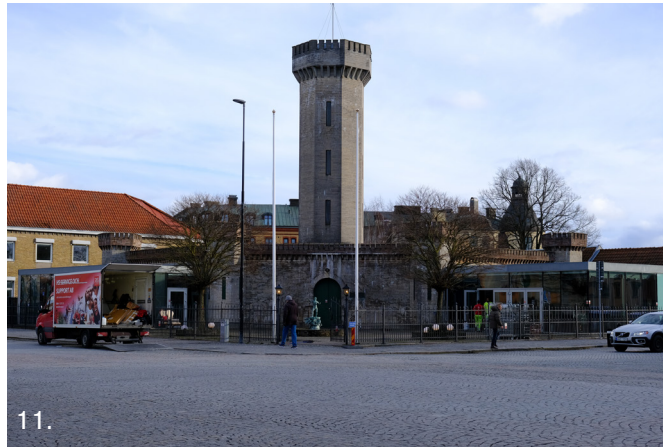
11. The Water Castle Built in 1863 in a French Normandy castle style to accomodate the water supply problem the city struggled with since its founding. The façades are clad with limestone. Additions were made in 2008 when the property was redesigned to be a restaurant/art gallery. The building is nationally listed and has a well preserved exterior, apart from the additions.
