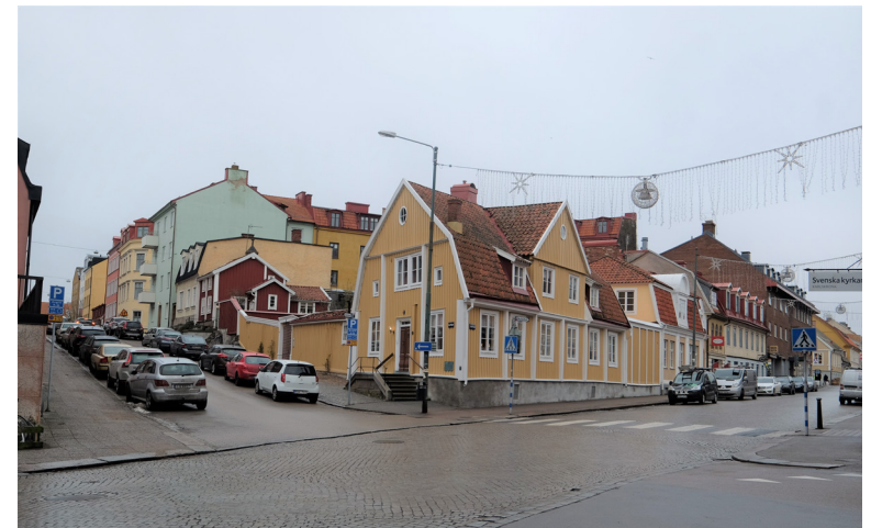
The corner building on the block Rådmannen. The sharp angle visualizes the original city plan and its diagonal streets cutting through the grid plan. The building is nationally listed.
