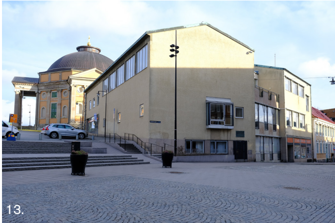
The City Library Built in 1959 in a characteristic Swedish 1950's style; the modernist principles about form following function combined with a higher grade of detailing and variation in the architectural expression. The façades are clad with plaster and marble. Well preserved exterior and interior.
