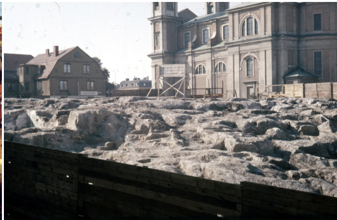
The Hjulhammar block after demolition 1959-08-14.
