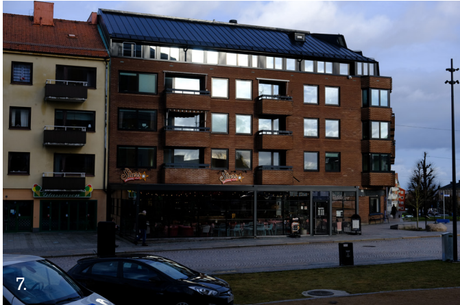
7. Sheldon 1 Sheldon 1 is an apartment building built in 1972. Replaced a neo renaissance building from the 1890's. Generally well preserved exterior.
