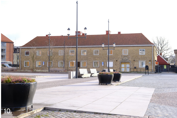
10. Former Post Office Built in 1942 in a neo realist style. Replaced two wooden houses from 1790. Rebuilt in the 1980's. Façade towards the square is generally well preserved, other façades altered. Interior remodeled entirely.
