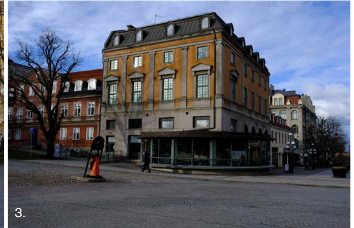
3. Magistraten 16 Built in 1901 in an Art Nouveau/Neo Rococo style. Rebuilt in the 1920's in a Neo Baroque style. Minor additions towards the square from the 2000's. Generally well preserved exterior from the 1920's.
