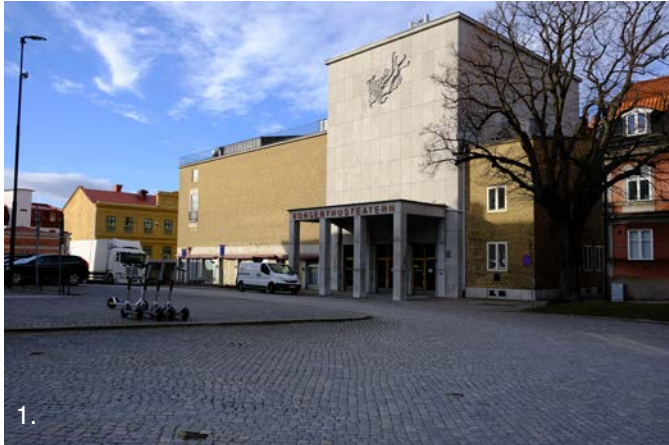
1. Concert house Built in 1939 in a modernist style, consisting of two rectangular blocks, clad in yellow brick and marble. Built on a plot where the previous buildings were destroyed in the city fire of 1909. Well preserved exterior.
