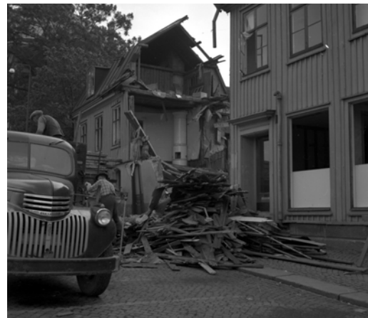
A wooden house from 1790 is being demolished to make way for the new City Library in 1957.
