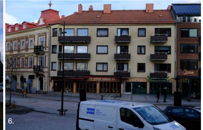
6. Sheldon 29 Sheldon 29 is an apartment building built in 1942. Replaced a wooden house from 1790. Exterior has undergone distorting changes.
