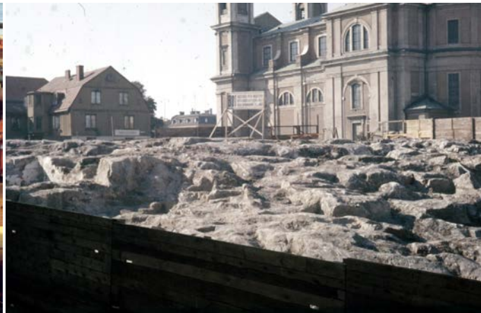
The Hjulhammar block after demolition 1959-08-14.
