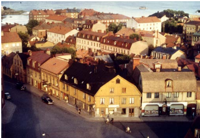
The Hjulhammar block before demolition, 1950's.
