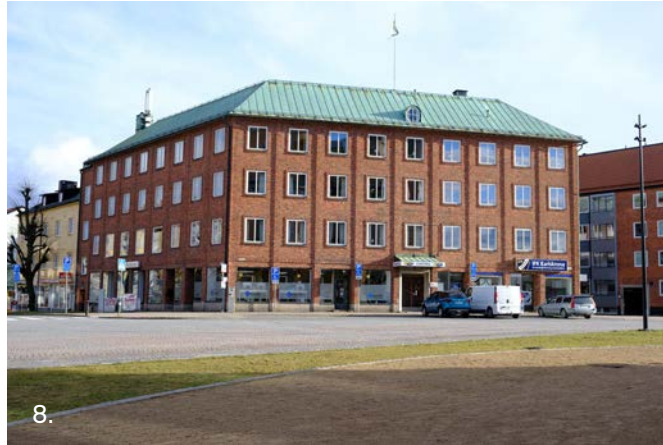
8. The Military home Built in 1951 in a neo realist/neo classicist style, yet still unmistakably built in the 1950's. Façade in brick, slated roofs covered with copper. Replaced three wooden houses from the 1790's and one brick hous from the 1800's.
