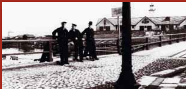
The Stumholmen Bridge “The Bridge of Sighs”
